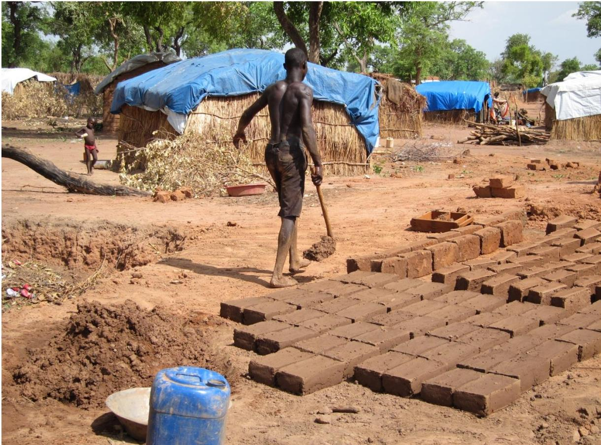
**Fig. 5.** Use of mud bricks for shelter construction in Yida settlement
